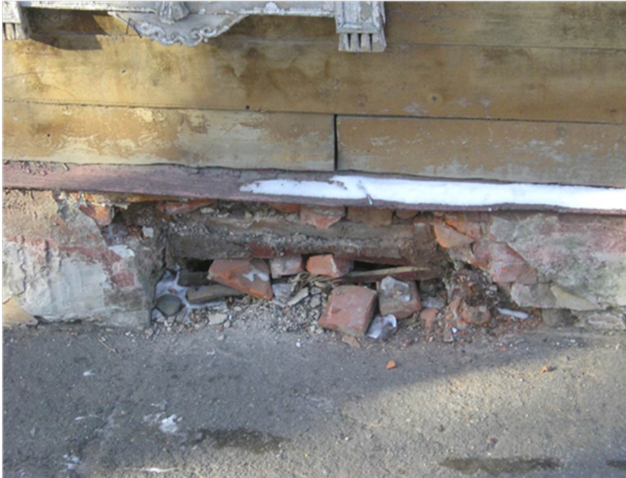
Fig. 2. Condition of the basement part of the walls
