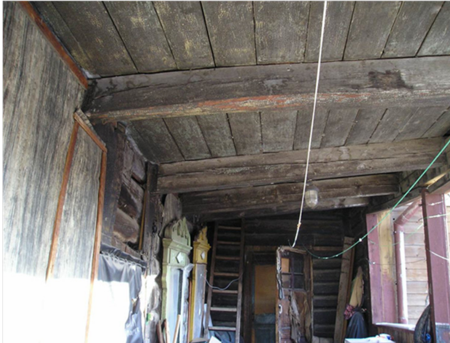
Fig. 6. The condition of the floor beams
