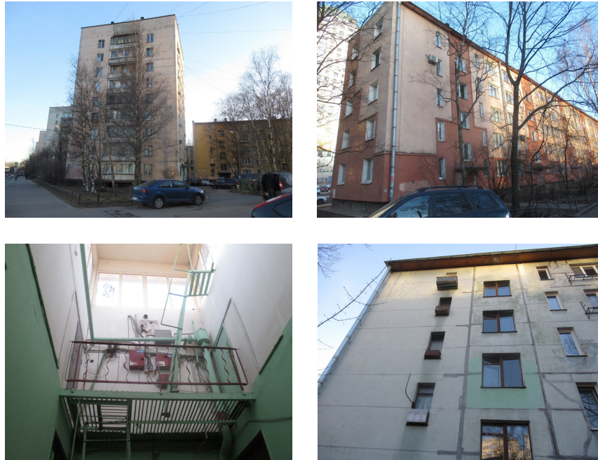
Fig. 3. An ensemble of panel blocks at the corner of Narodnogo Opolcheniya Avenue and Leninsky Prospekt in Leningrad: a) point 9-storey houses of the G-5i series; b) linear 5-storey house of the G1 series on Narodnogo militia avenue; c) skylight and utilities; d) part of the courtyard facade
